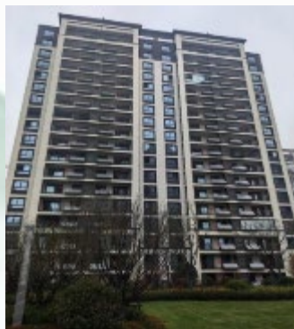
Solar Water Heaters
