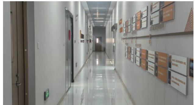
Upgrading of the central control room at Cangzhou Power Plant of the North China Region
