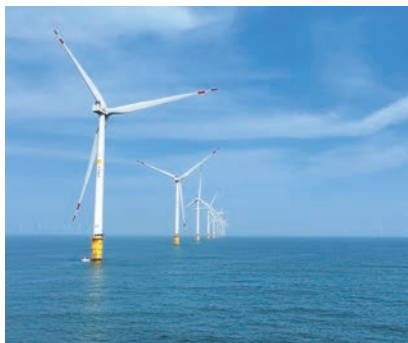
In January 2023, the Zhejiang Cangnan #1 400MW Offshore Wind Power Project achieved full-capacity grid connection
