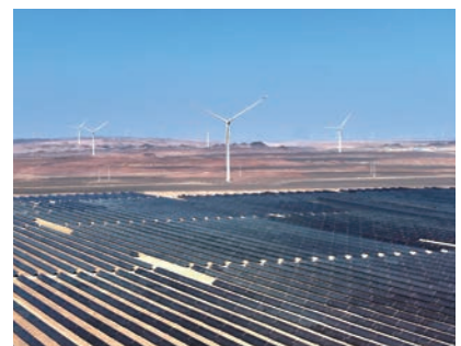
In December 2025, the 4,000MW Renewable Energy Project at Chongqing Energy Xinjiang Tianshan Northern Foothills Renewable Energy Base was completed and connected to the grid
