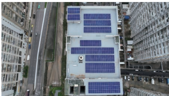
CR Power's 230kWp Distributed Photovoltaic Power Project at Shatin Warehouse in Hong Kong achieved full-capacity grid connection in August 2025
