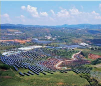
In March 2023, the Yunnan Yiliang Xinfa 120MW Medicine-Solar Hybrid Photovoltaic Power Generation Project achieved full-capacity grid connection
