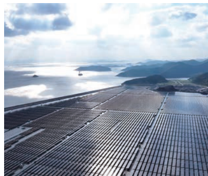
The 250MW Zhejiang Daishan Shuangjiantu Tidal Flat Centralized Fishery-Solar Hybrid Power Station achieved grid connection for Phase I (September 2023) and Phase II (December 2024) respectively
