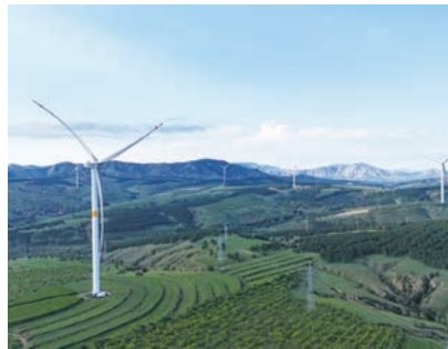
In December 2024, the Liaoning Chaoyang Shaoguoyingzi 300MW Wind Power Project achieved full-capacity grid connection
