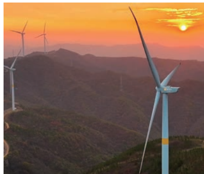
In December 2024, the Hubei Hong'an Tianming 150MW Wind Power Project achieved full-capacity grid connection
