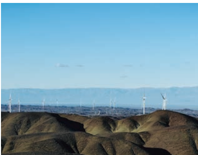
In October 2024, the Santanghu 1,000MW Wind Power Project achieved full-capacity grid connection
