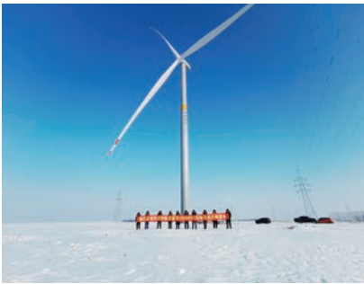
In December 2023, the Heilongjiang Jiamusi Fujin 150MW Wind Power Project achieved full-capacity grid connection
