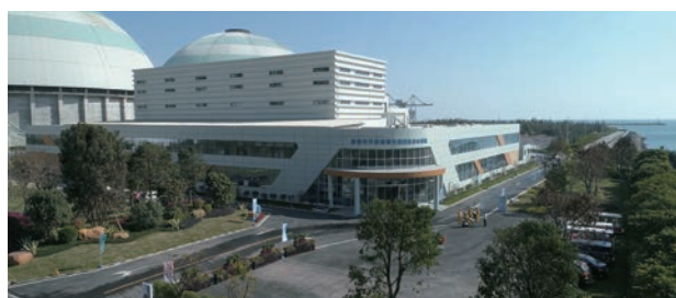
Shenzhen Ecological Demonstration Park for Sludge-to-Energy Utilization
