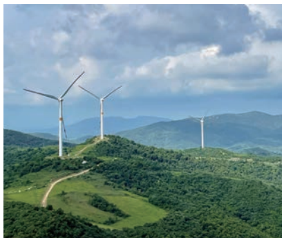
In February 2023, the Shaanxi Tiancheng 100MW Wind Power Project achieved full-capacity grid connection
