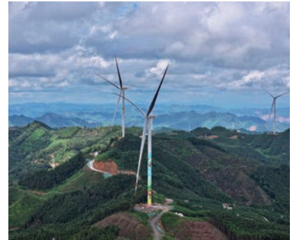
In December 2024, the Guangxi Baise Tianlin Badu 200MW Integrated Wind Power and Energy Storage Project achieved full-capacity grid connection
