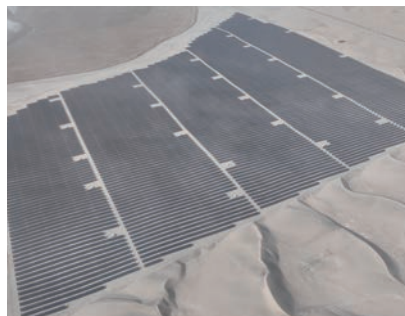
In May 2025, the Hotan 500MW Photovoltaic Desertification Control Project achieved full-capacity grid connection
