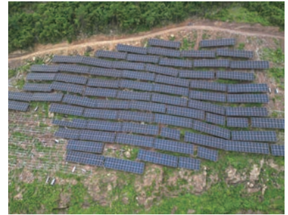
In December 2025, the Chongqing Yunyang Gaoyang 65.6MW Photovoltaic Power Project successfully completed inverse power transmission in a single attempt
