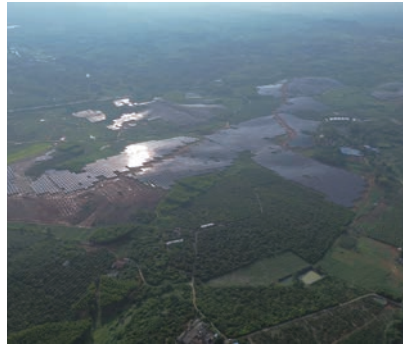
In December 2024, the Guangxi Nanning Wuming 300MW Integrated Agriculture-Photovoltaic-Energy Storage Photovoltaic Power Generation Project achieved full-capacity grid connection
