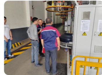
Electrical Safety Hazard Inspection
