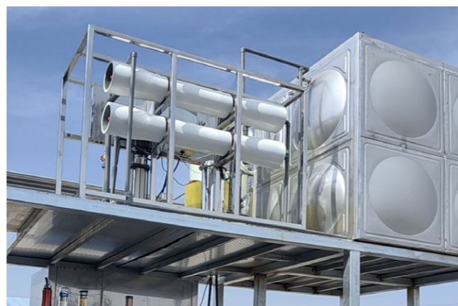
· Wastewater Reuse System for Dairy Parlor Equipment ·
