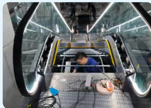
Elevator Renovation Site
