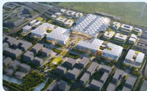
Energy Center of Shanghai East Railway Station, Eastern Hub
