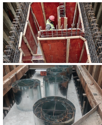
Facility Construction Site
