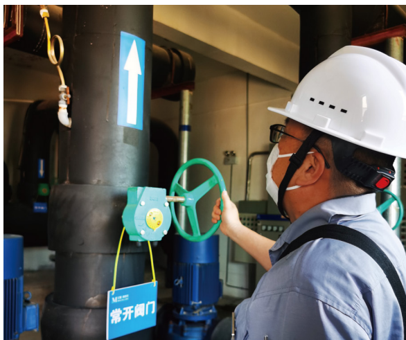
Routine Inspection of Daily Water Supply Facilities
