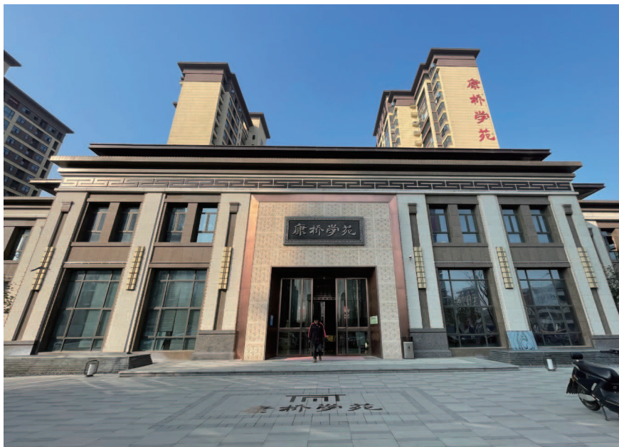
The Xixian Kangqiao Xueyuan project in Henan Province
