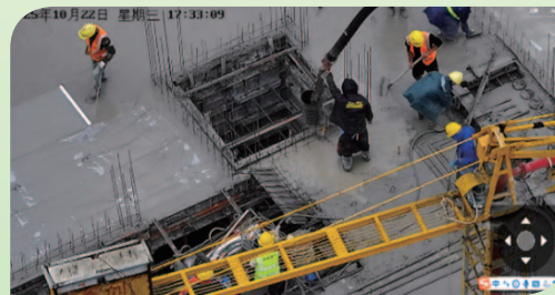
“Skynet” inspecting concrete pouring for floor slab
