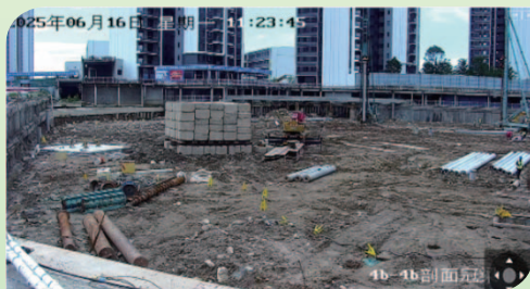
“Skynet” inspecting pile foundation construction and excavation safety on-site
