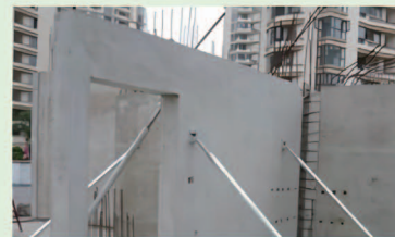
Prefabricated wall panels
