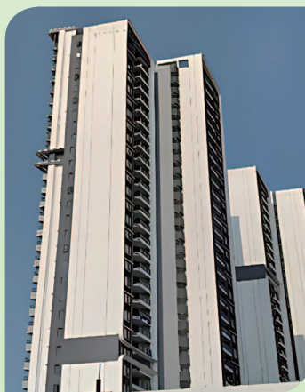
Agile North Tower Project (Awarded Provincial Quality Structure Award)
