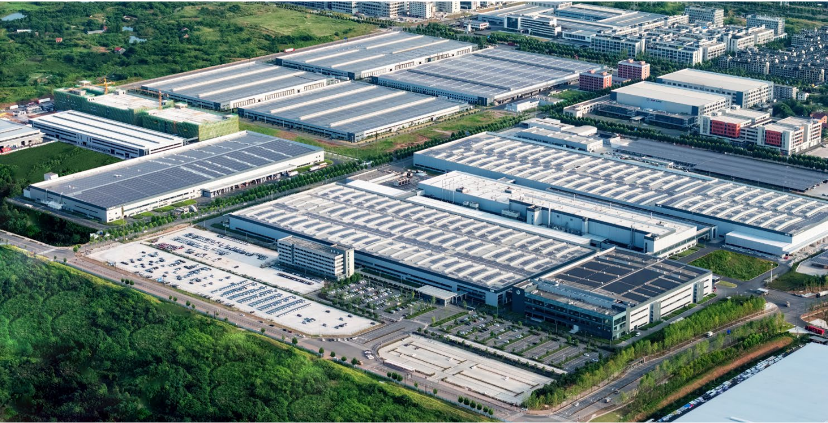
PV system installation at Leapmotor facilities
