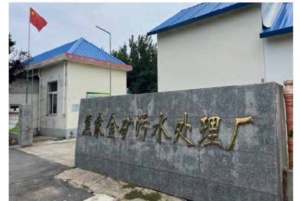
Jiaojia Gold Mine Domestic Sewage Treatment Plant
