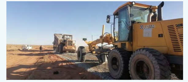
Changtai Mining Dispatched a Disaster Relief Team to Repair the Road
