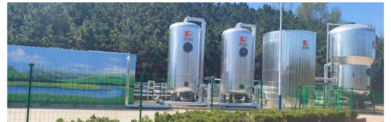
Guilaizhuang Gold Mine Water Purification Project
