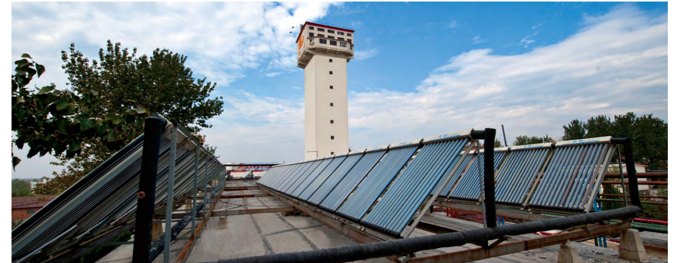
Jiaojia Gold Mine Laying Photovoltaic Panels
