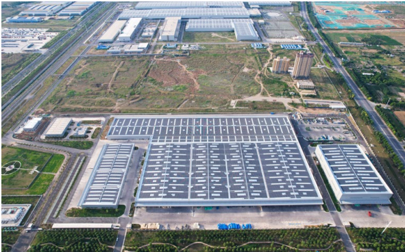
Laiwu Factory Distributed Photovoltaic Power Station
