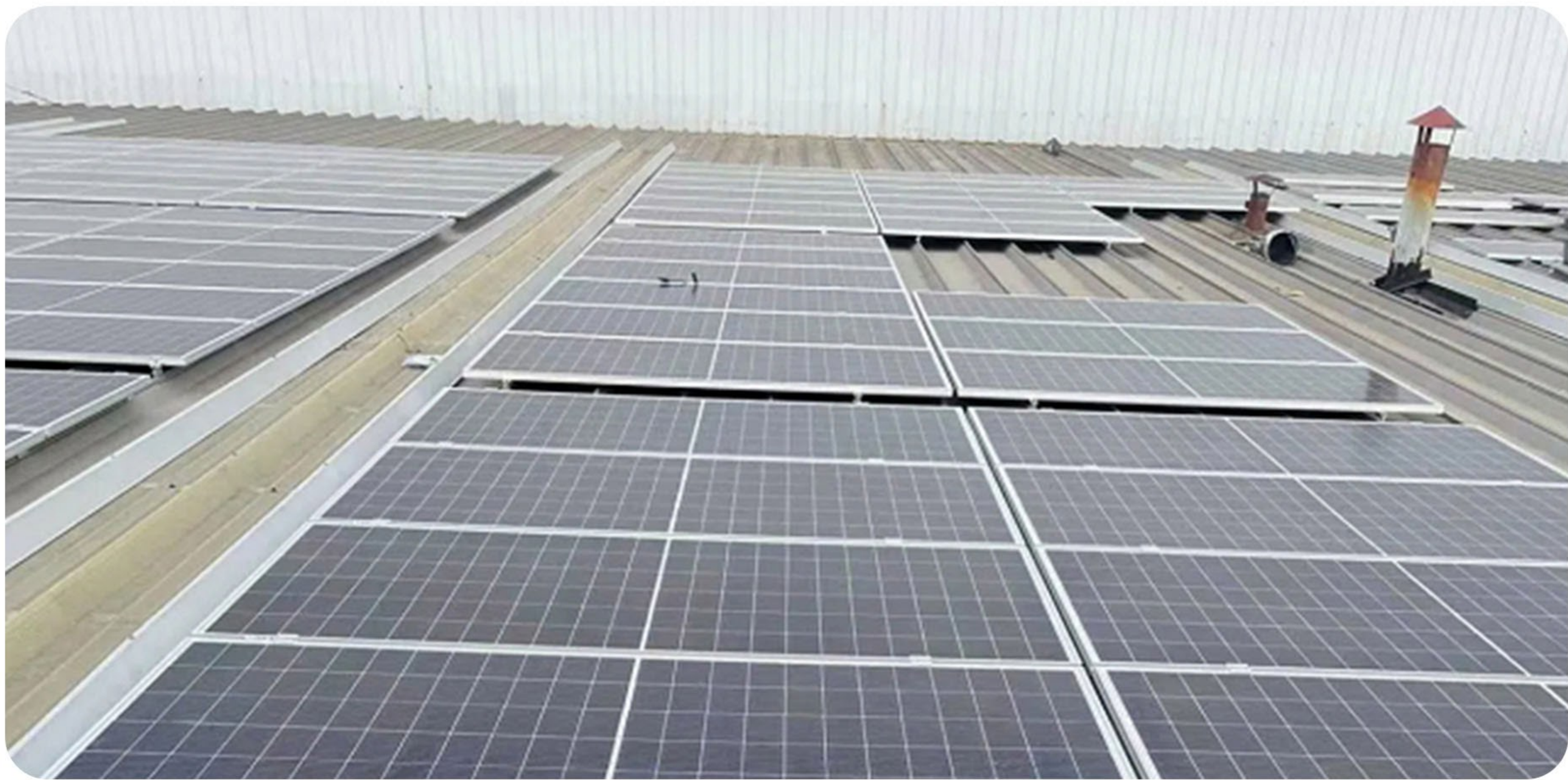
Installation of photovoltaic systems
