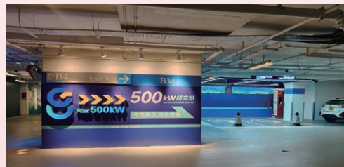
圖：「充美好」超充站 Picture: “Chongmeihao” Ultra-Fast Charging Station
