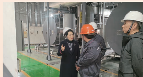
圖：無錫區域檢查 Picture: Inspection in Wuxi Region
