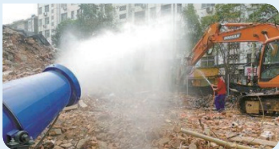
Site dust control: fog cannon
