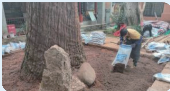
Example of soil improvement
