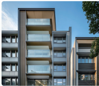
Nearly zero energy project: Shanghai Yangpu Tianyue
