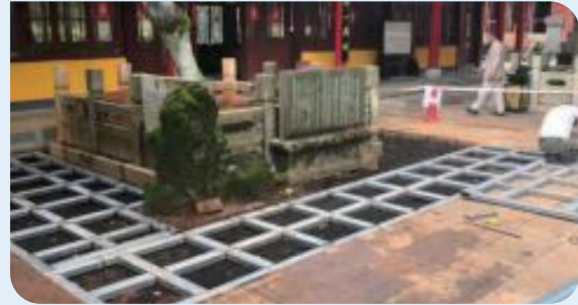
Keel platform welding
