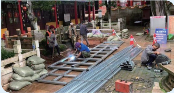
Keel platform welding
