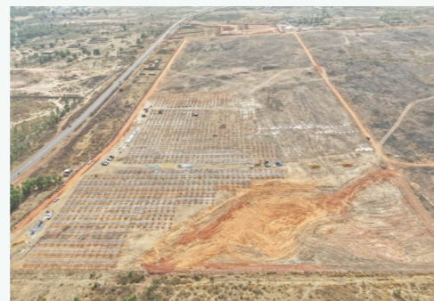
Construction site of the Mali integrated solar-energy storage power station
