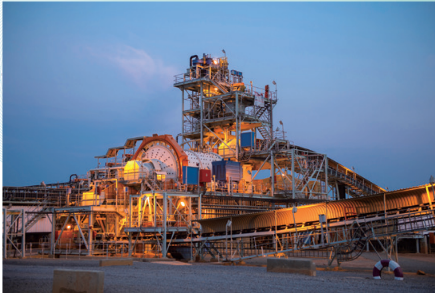
Kinsenda Mine – Processing Plant Kinsenda礦場 — 選礦廠
