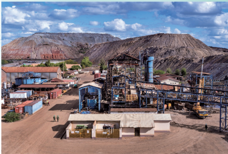
Ruashi Mine – Processing Plant Ruashi礦場—選礦廠
