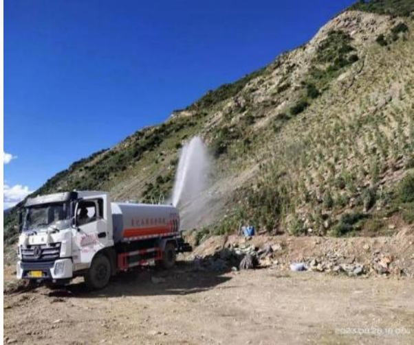
Slope Tree Planting Operations
