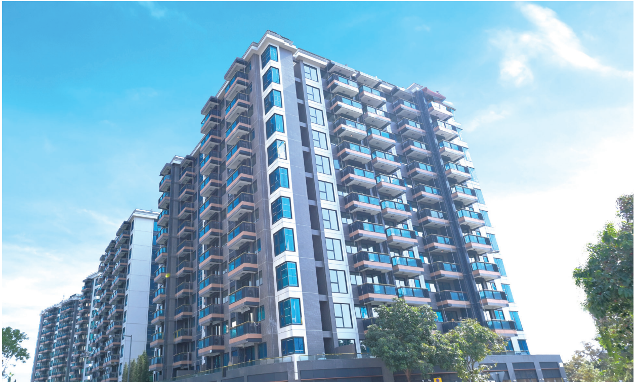
Residential development “ High Park ” in Hung Shui Kiu
