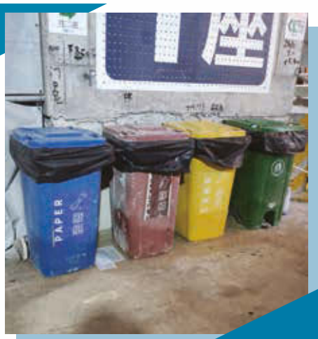
▶ Variety recycling bins are placed on construction sites 於建築地盤放置多種回收箱
