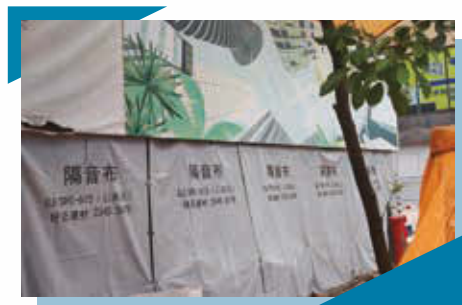
Noise barriers hang on the hoarding 於圍板繫上隔音屏障
