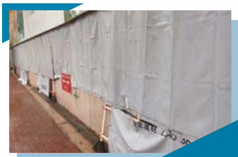
Noise barriers hang on the hoarding 於圍板繫上隔音屏障
