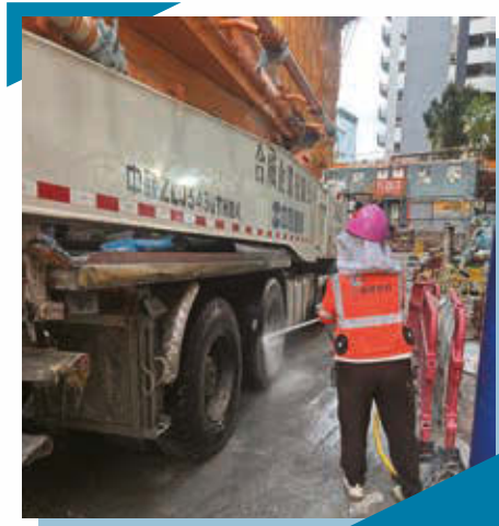
Designated wheel washing area at site 於地盤設立指定輪胎清洗區
