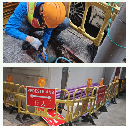
Street Lighting Circuit Improvement Works in Kowloon City District
