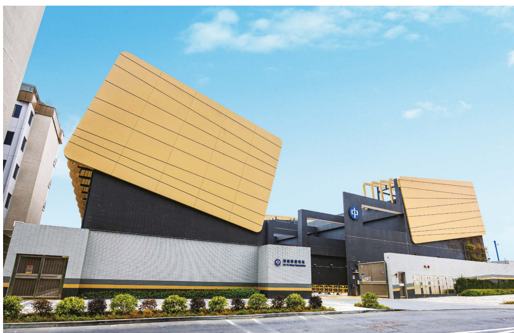
Ho To West Substation in the Northern Metropolis is part of CLP's timely investments to strengthen Hong Kong's power system and support the city's next phase of growth.
