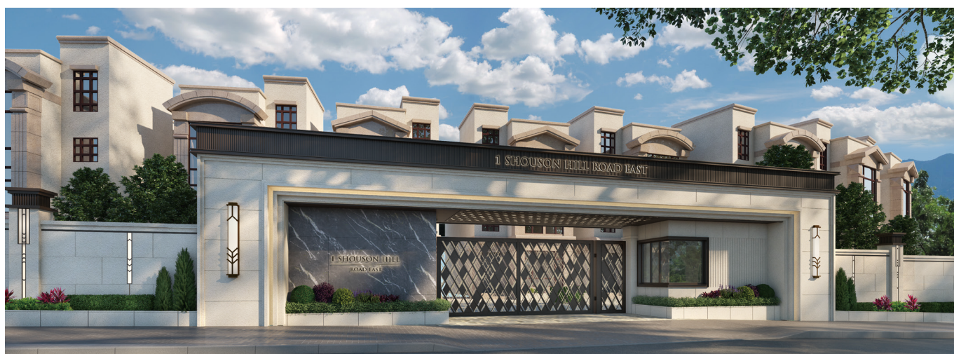
1 Shouson Hill Road East, Hong Kong
