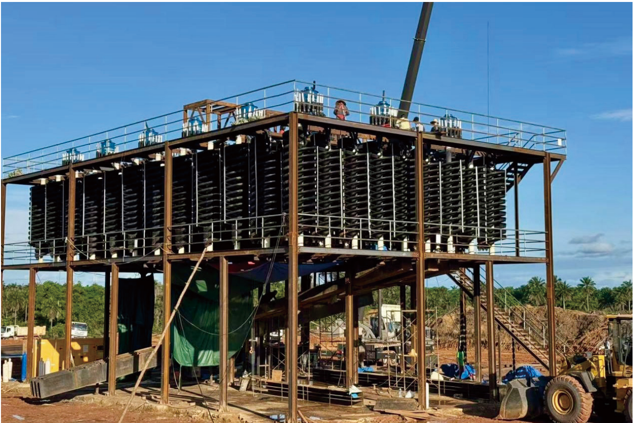
Official Commencement of Operations of the First Production Line of the Rutile Project
