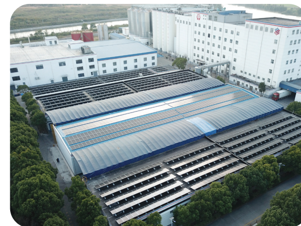
The 0.7-MW solar PV modules installed in the flour mill in Jintan
