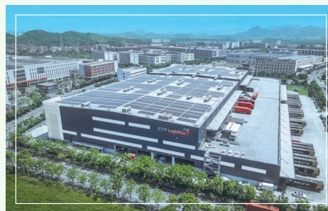
The rooftop solar PV system in East China
